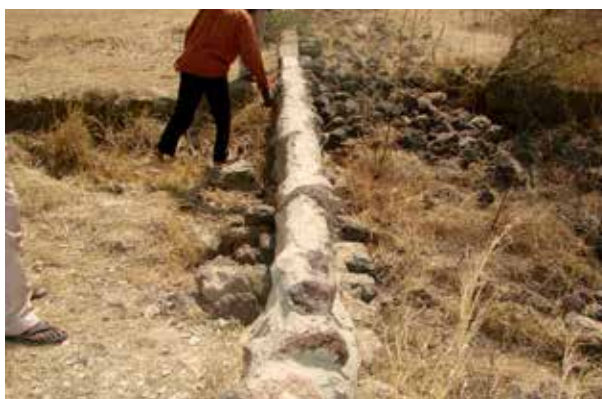
Repairs made by Sisené to Basin
